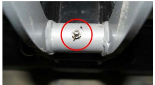
Fig. 17: Bolt in bottom of main boom.
